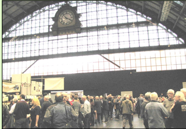
A reminder that the venue was once a magnificent station for the old Central Railway
